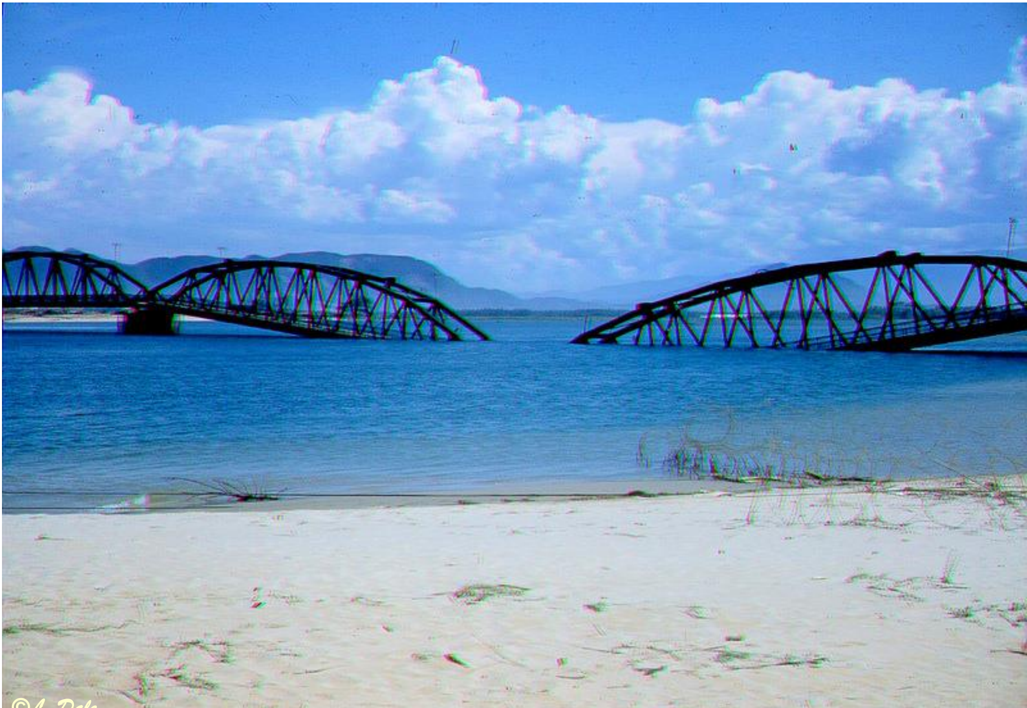
The dropped spans of the Nam O Bridge
